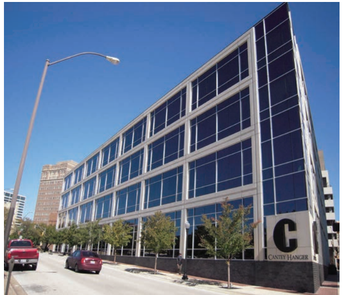
CANTEY HANGER BUILDING Cantey Hanger is a 4-story, 35,000 square foot, mixed use building located in downtown Fort Worth, Texas.
